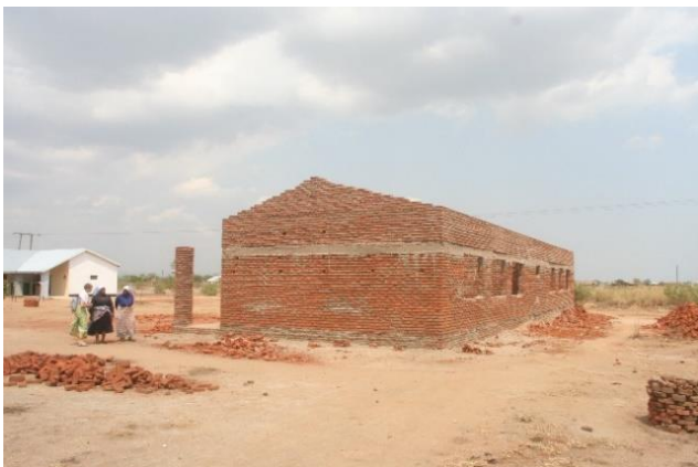
Foto 1: school in aanbouw november 2019
