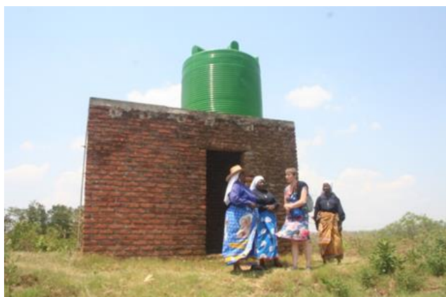
Foto 3: waterpomp met reservoir (november 2019)
